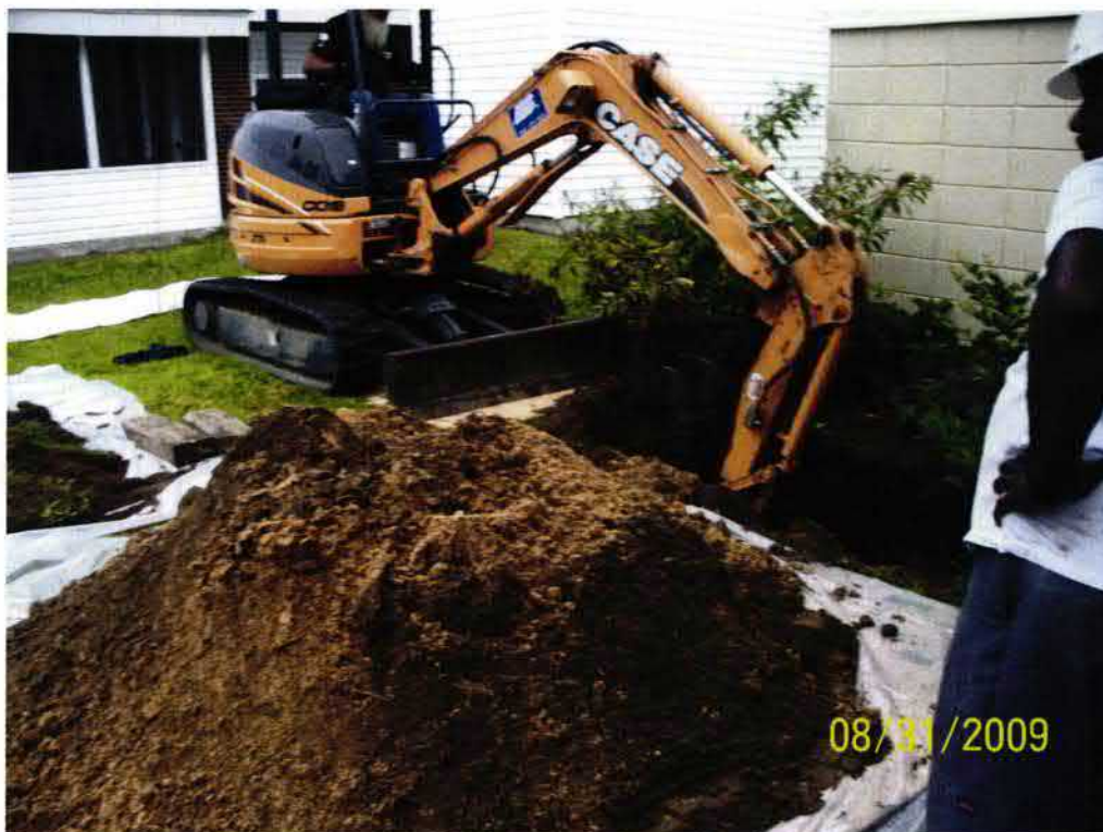
Picture 2: UST 1246Dove removal in progress.
